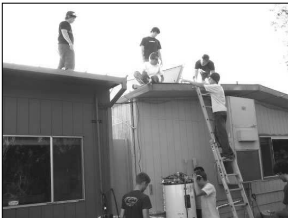
Figure 6. A team of freshmen design and build a solar water heating system for a local elementary school and science museum to enable young children to wash their hands with warm water and to provide an exhibit to learn about solar power.
